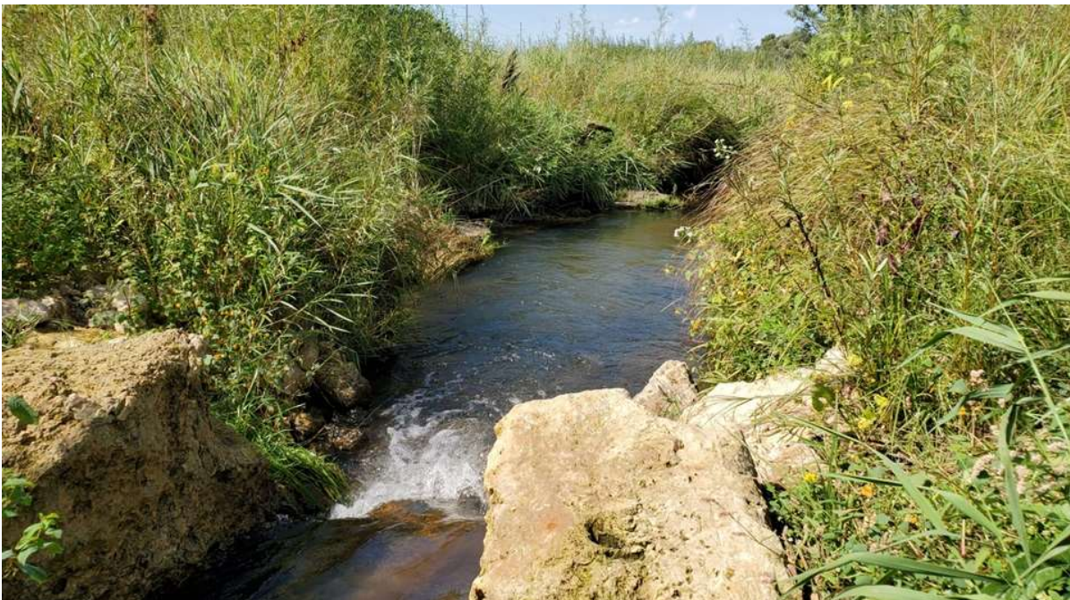
A year after installation, the ERO has scoured approximately 9 cubic yards of sand.
